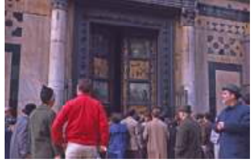
Damaged Baptistry doors and fallen Ghiberti panels, Piazza San Giovanni
